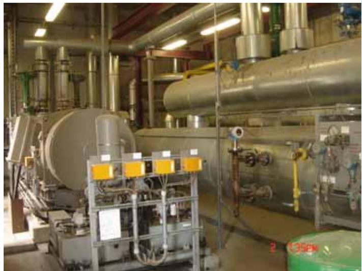
The installation of organic Rankine cycle at Heidelberg Cement, Lengfurt has been the first of its kind in the cement industry. For the cement production capacity of 1.0 MTPA at Lengfurt, the waste heat recovery based power generation is rated for a capacity of 1.5 MW. The net power export to the cement plant, after accounting for the auxiliary power consumption in the power house, is 1.3 MW.
